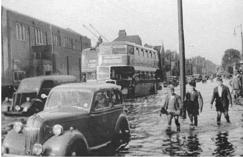
The River Lea and linked channels flow through the Olympic Park. Description of the risk and solution:
